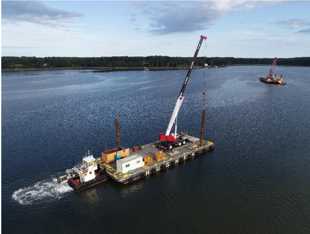
Figure E-7. Assist barge being moved into position by 650HP tug for an anchor change. 5:02 PM, Sept 9, 2019.
