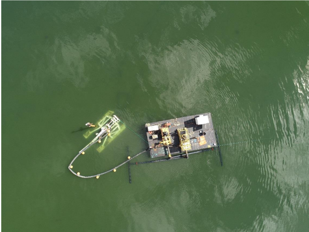
Figure E-1. Stationary jet plow in position with pump barge, prior to start of jet plow. 11:52 AM, Sept 9, 2019.
